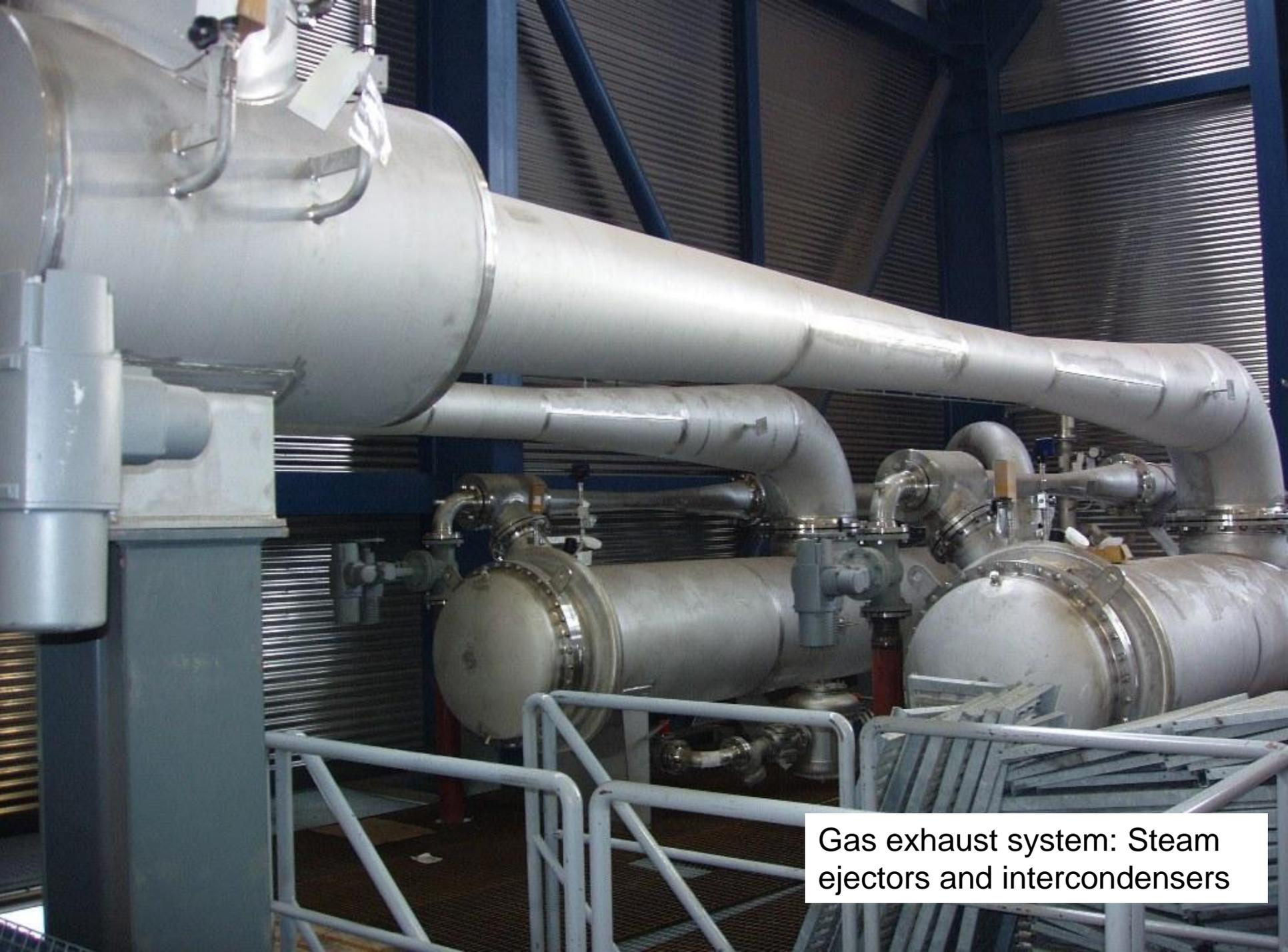
Gas exhaust system: Steam ejectors and intercondensers
