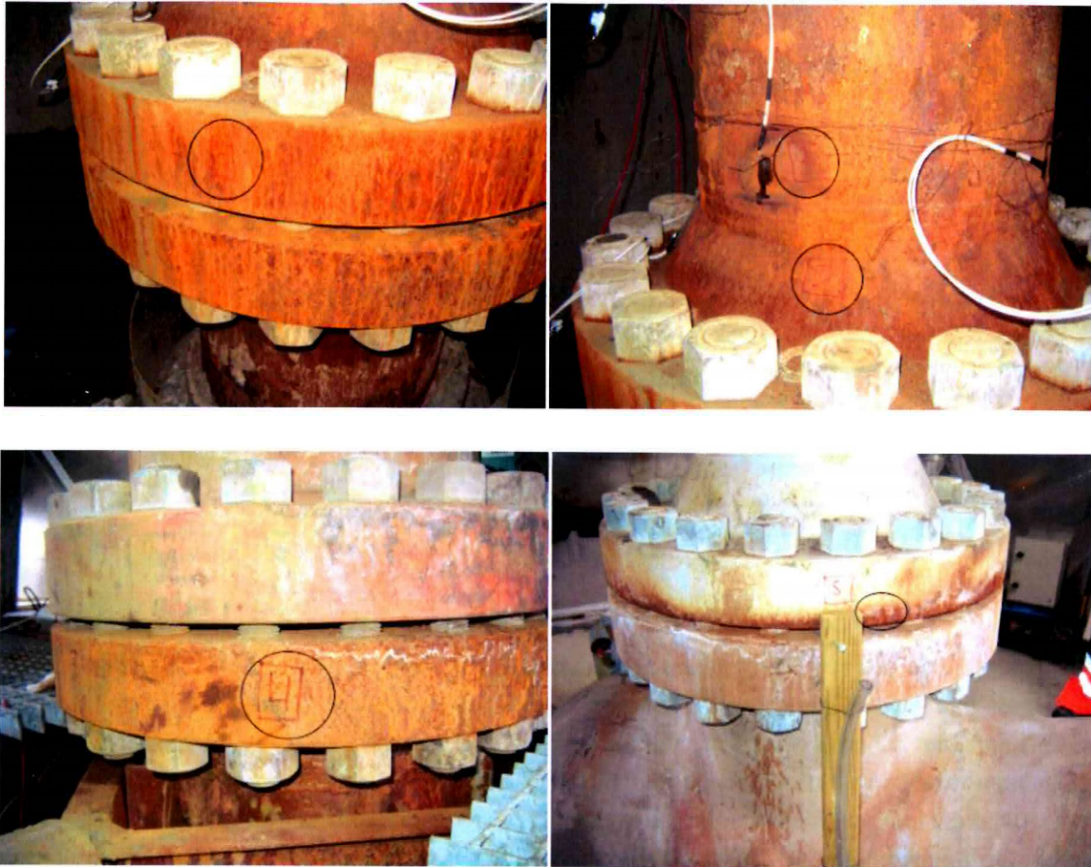
Figure A.4 Location of temperature measurements on wellhead HE-46
