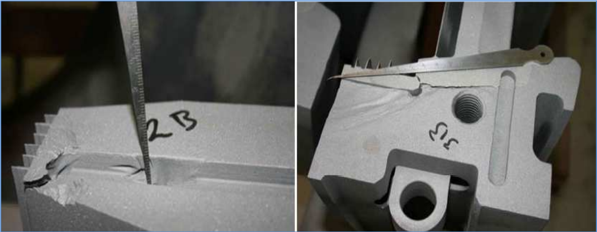
Figure 4.7 Left, erosion damage on the horizontal joint on the second stage diaphragm in turbine 2 at Hellisheiði power plant. Right, erosion damage on the horizontal joint on the third stage diaphragm in turbine 3 at Hellisheiði power plant [41].
