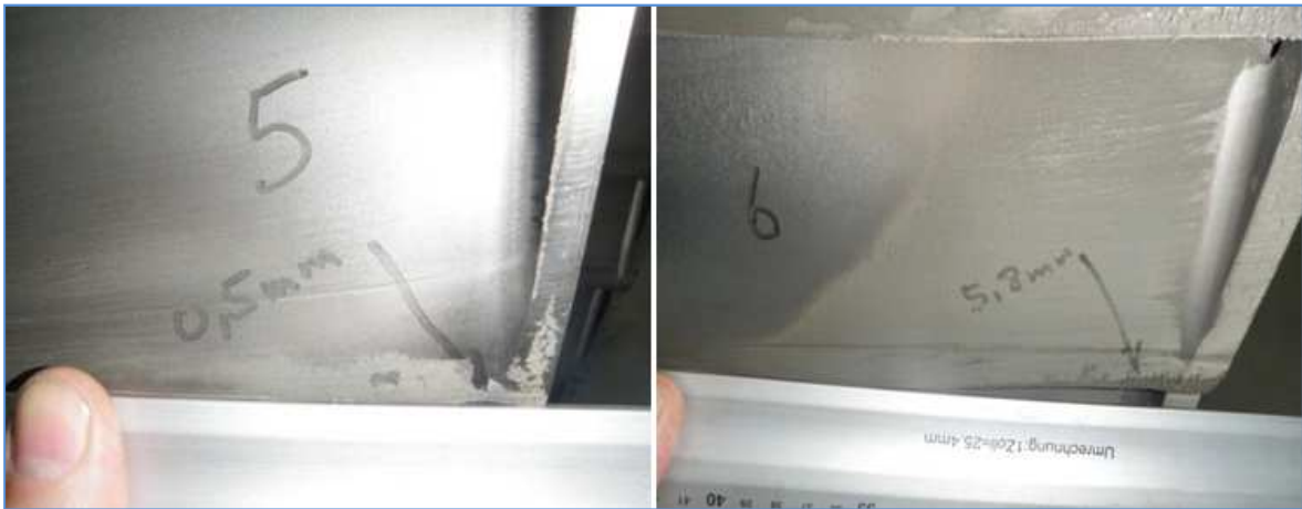
Figure 4.17 Both pictures are from turbine 1 at Hellisheiði power plant. Left, material deterioration at a fifth stage rotor blade. Right, material deterioration at a sixth stage rotor blade [41].
