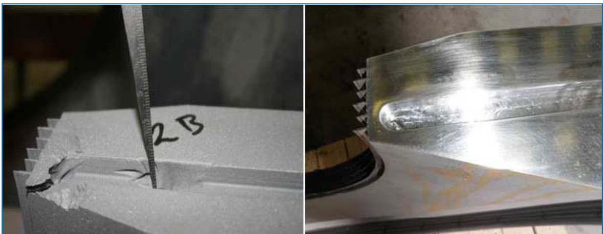
Figure 4.22 Both pictures are of the horizontal joint on the second stage diaphragm in turbine two at Hellisheiði power plant. Left, the horizontal joint before repair. Right, the horizontal joint after repair [41].
