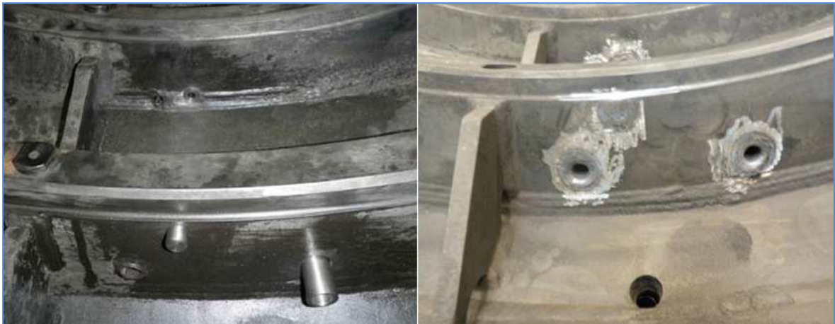
Figure 4.31 Left, drain holes in a diaphragm attachment in turbine two at Hellisheiði power plant with stainless steel cylinders fitted in. Right, drain holes in a diaphragm attachment in turbine one at Hellisheiði power plant after being repaired with stainless steel cylinders [41].
