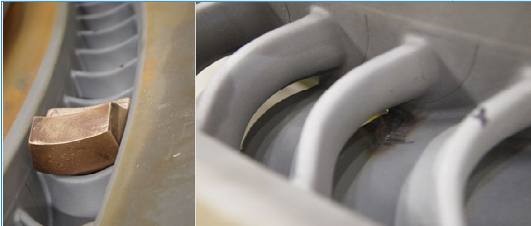
Figure 4.25 Left, cooling element to cool stator blades on a diaphragm during welding. Right, the stator blades on the first stage diaphragm in turbine 3 at Hellisheiði power plant after welding.
