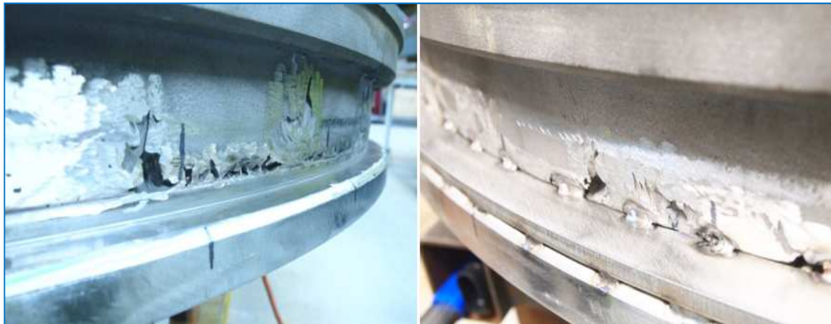
Figure 4.23 Both pictures are of a diaphragm from a steam turbine at Nesjavellir power plant. Left, wear in a casing seat, the side of the seat has been milled down. Right, here a piece of stainless steel is being welded over the side of the casing seat.
