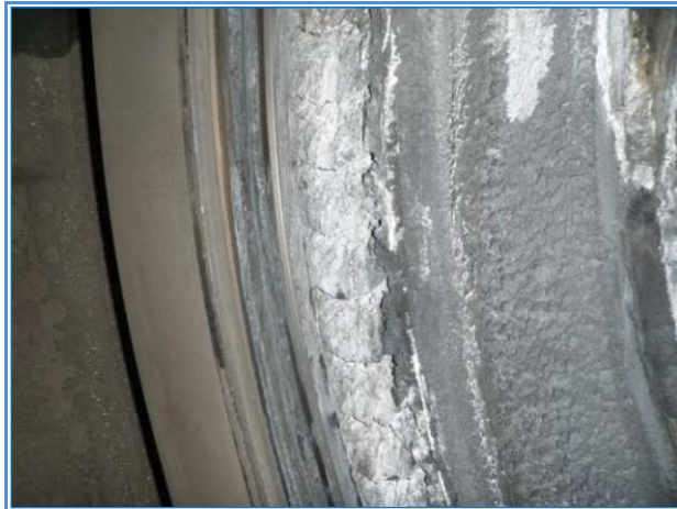
Figure 4.3 Silica scaling on the first stage diaphragm in turbine 3 at Hellisheiði power plant [41].
