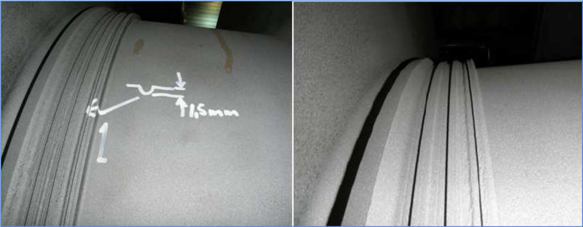
Figure 4.14 Left, 1.5mm wear of the rotor labyrinth seal for diaphragm two in turbine 3 at Hellisheiði power plant. Right, about 1mm wear of the rotor labyrinth seal for diaphragm two in turbine 2 at Hellisheiði power plant [41].
