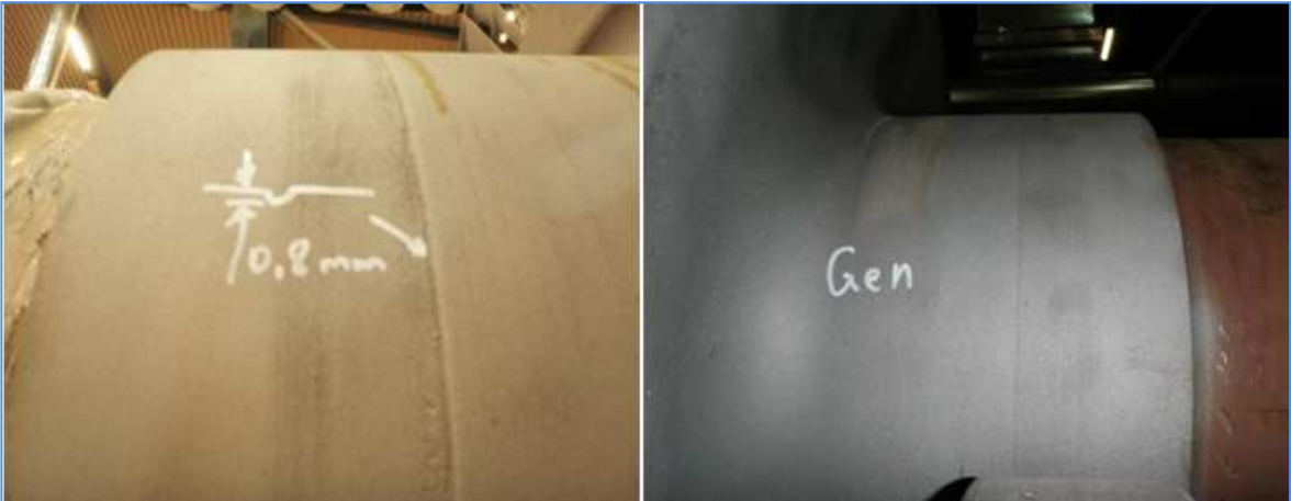
Figure 4.13 Both pictures are from turbine 3 at Hellisheiði power plant. Left, wear of the low pressure seal surface. Right, the high pressure seal surface, which has almost no wear [41].
