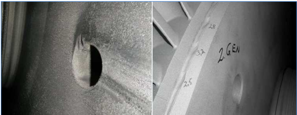
Figure 4.15 Left, wear of a steam balance hole at stage 3 in turbine 1 at Hellisheiði power plant. Right, wear at the backside of the rotor drum, beside the rotor blades roots at stage 2 in turbine 2 at Hellisheiði power plant [41].
