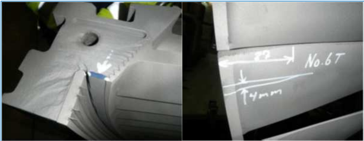
Figure 4.4 Both pictures are from turbine 3 at Hellisheiði power plant. Left, wear due to erosion on the horizontal joint on the fourth stage diaphragm. Right, wear due to erosion on the leading edge and the back face of the leading edge at the tip of a rotor blade at stage six [41].
