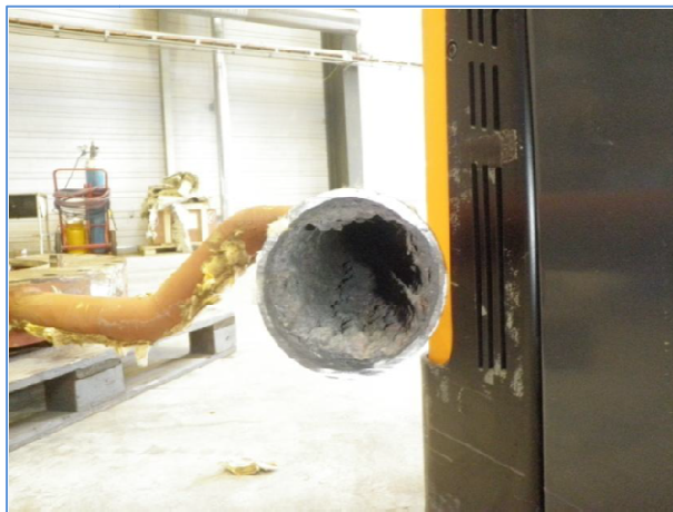
Figure 4.18 Scaling in the pipe, which transports the steam from the high pressure gland seal to a condenser, for the low pressure turbine manufactured by Toshiba at Hellisheiði power plant [41].
