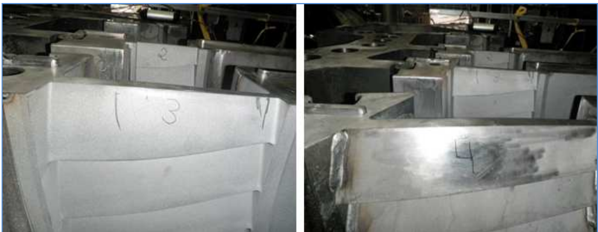
Figure 4.10 Both pictures are from turbine 3 at Hellisheiði power plant. Left, an example of the design of the inner and outer roots at the stator blades at stages 1-3 can be seen. Right, an example of the design of the inner and outer roots of the stator blades at stages 4-6 [41].
