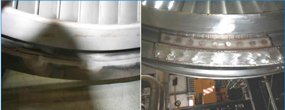
Figure 4.24 Left, the fourth stage diaphragm from turbine 2 at Hellisheiði power plant. Right, new diaphragm for the fourth stage in turbine 2 at Hellisheiði power plant with a shield to prevent erosion damage [41].
