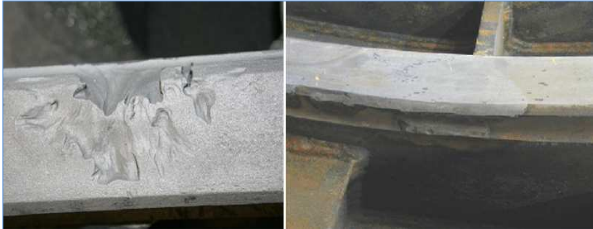
Figure 4.32 Left, wear at the diaphragm attachment in turbine two at Nesjavellir power plant. Right, diaphragm attachment in turbine two at Nesjavellir power plant after welding and polishing [41].
