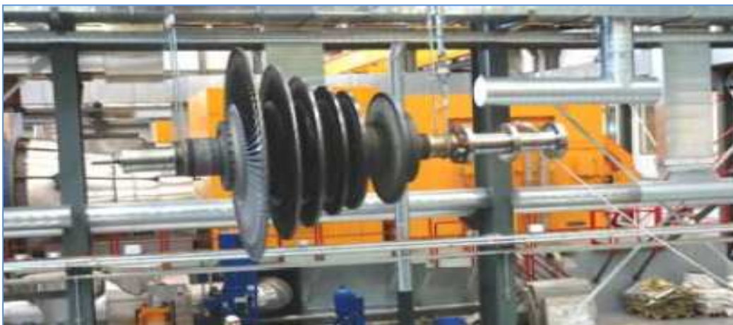
Figure 4.28 The rotor from turbine 2 at Hellisheiði power plant during overhauling of the turbine [41].
